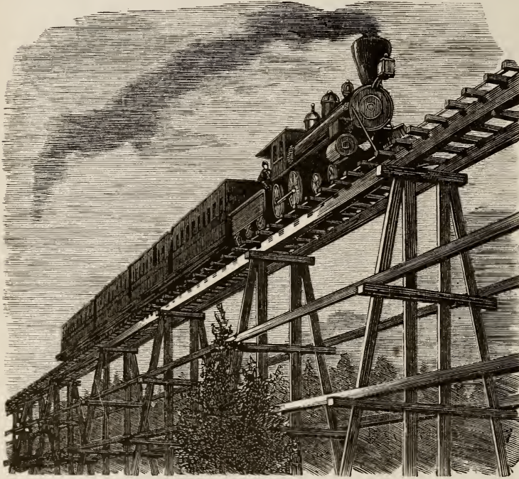
A TRESTLE ON THE NORTHERN PACIFIC.
